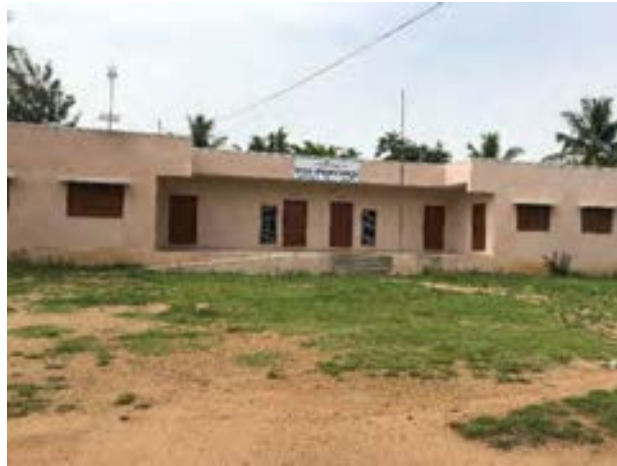
Ramp without railings, Government Highschool, Bannur, Hasan District
