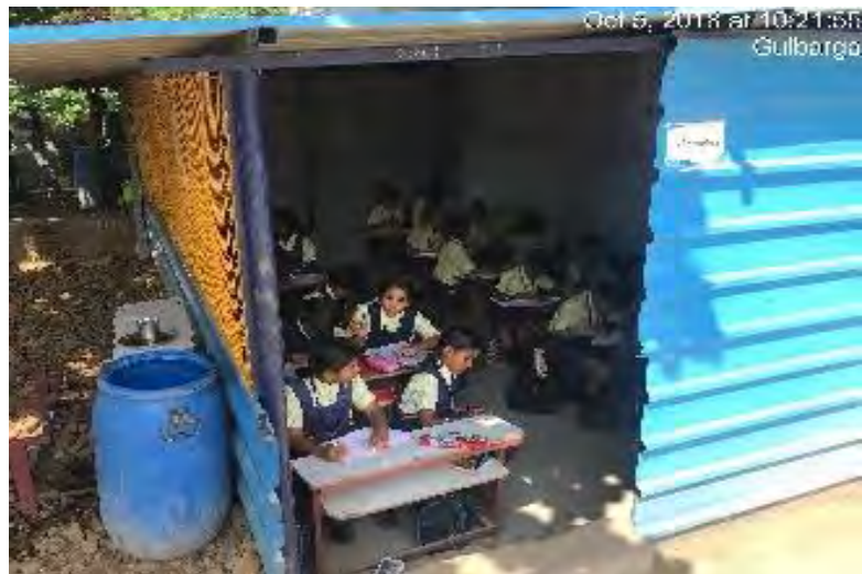
Sri Sai Central High School, Kalaburagi functioning in a structure made of asbestos sheet
